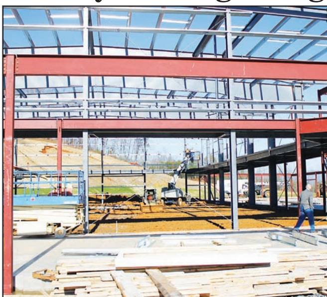
Commissioner Bill Kendall gets a close up view of construction of the county's new recreation facility. Photo/Libby Shook
