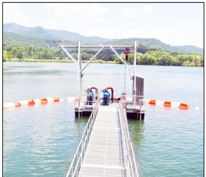
The City of Hiawassee's new water intake. It saves taxpayers' dollars. Of the remaining $600,000 for the cost of the projects, Hiawassee was able to get a low interest loan for
