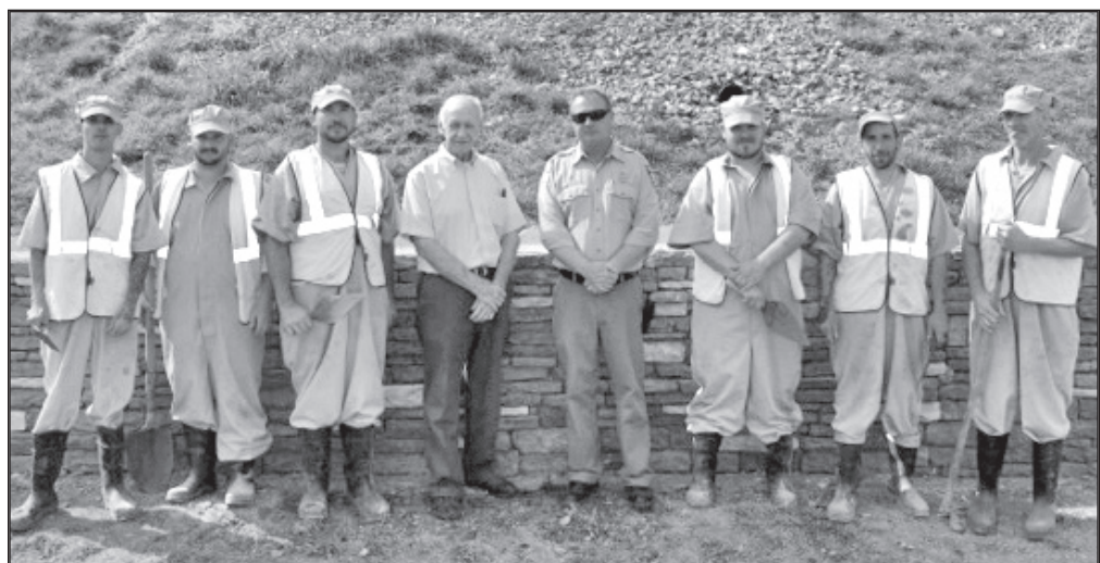
Commissioner Bill Kendall, Guard Cecil Shook, and county detainees were all satisfied with the way the wall has turned out
