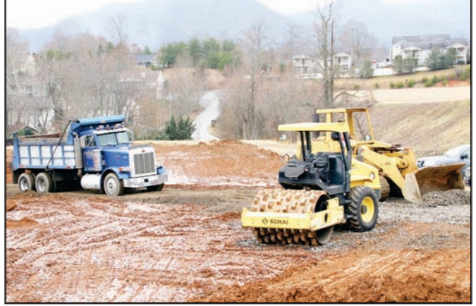
Grading is underway at the Taco Bell site. Photo/Shawn Jarrard
