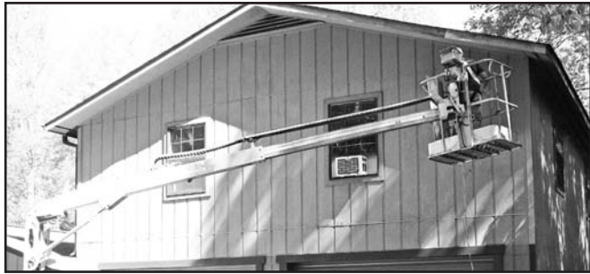
Brian Hollingshead sprayed part of the second floor of Station 3 in the cherry picker and Bob Garrett sprayed part.
