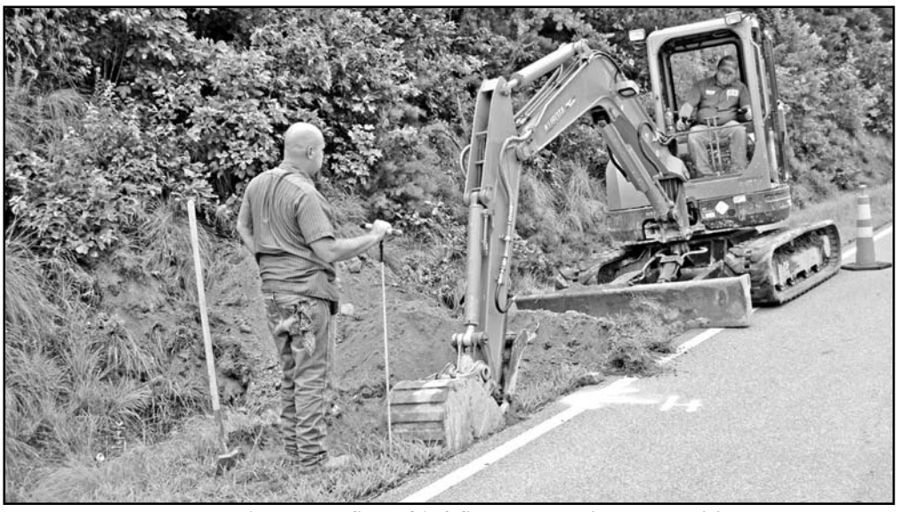
Work began last week to install the first of 150 fire hydrants in communities throughout the county to help lower the county's ISO fire rating to aid local homeowners. Photo/Lowell Nicholson
