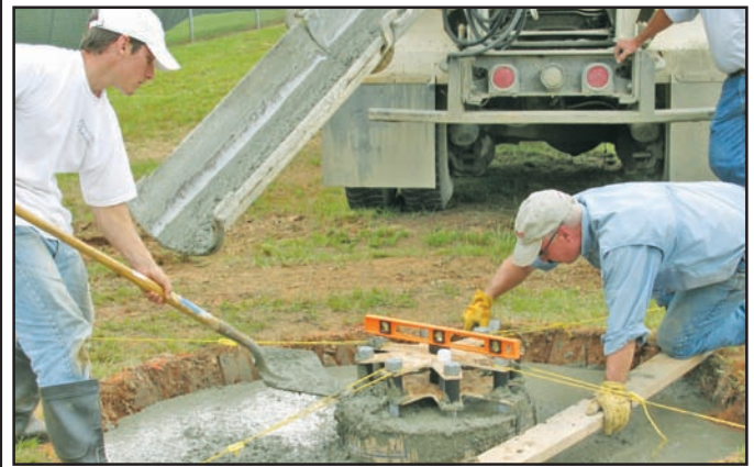
Workers complete phase I of the turbine project. Photo/Beth Wood
