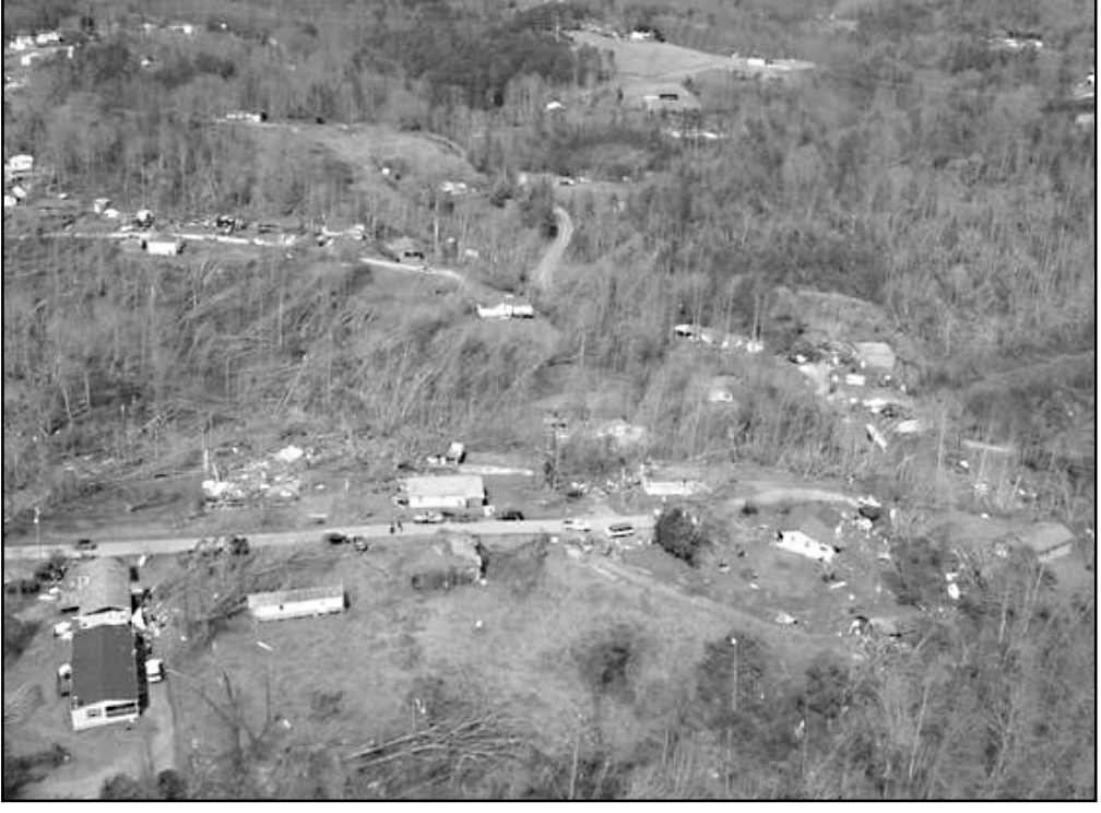
An aerial view of the Texana community along Joe Brown Road. This area endured its share of the wrath of an EF-2 tornado on March 2. Some homes were just lifted up and turned around.
