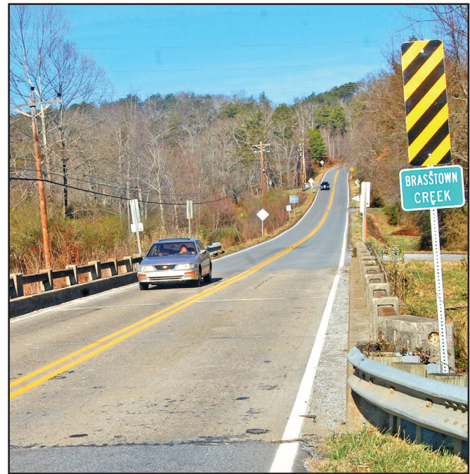
Brasstown Creek bridge, built in 1940, is scheduled for an upgrade in 2015, according to GDOT. Photo/Lowell Nicholson
